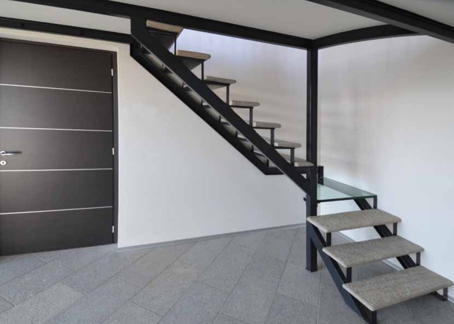
Scala in Luserna granigliata Scratched Luserna staircase
